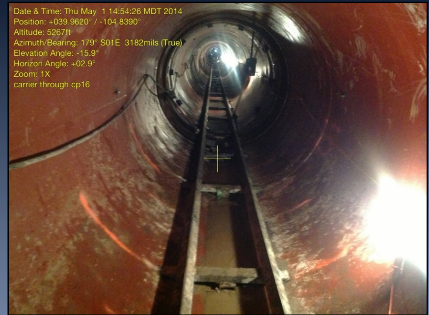
South Platte Interceptor construction tunneling equipment
